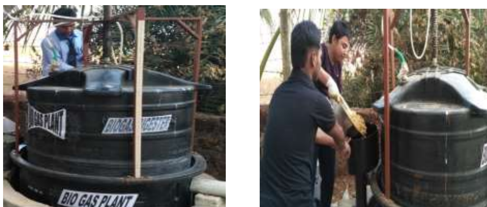
Fig 2 Biogas plant set up feeding slurry
